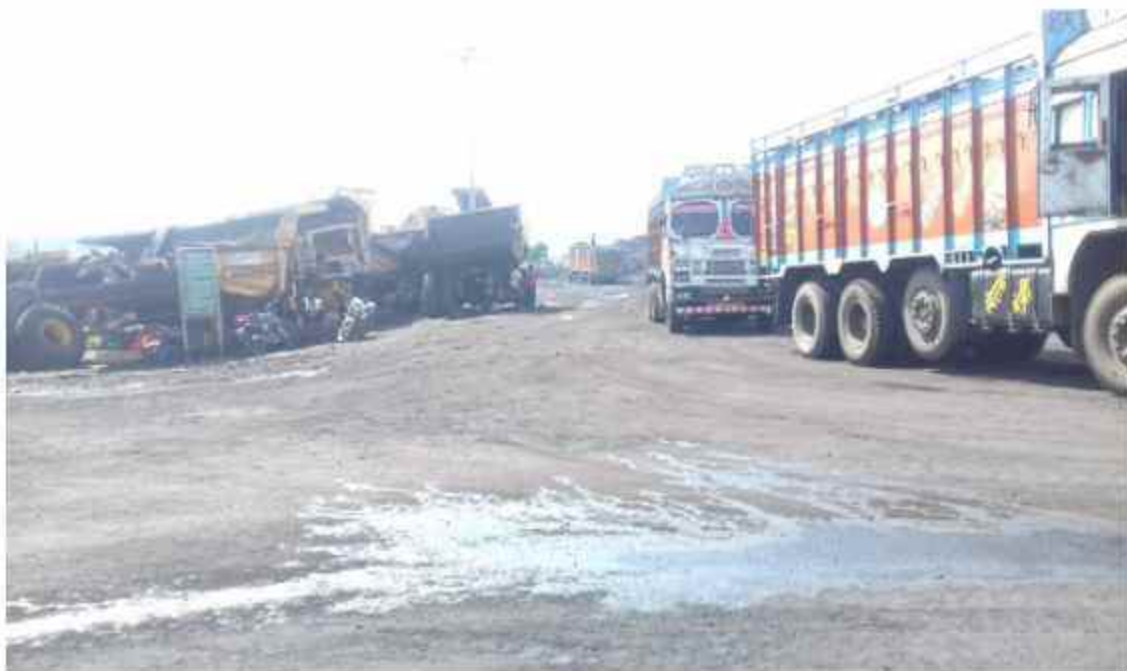
Roads constructed within colliery premises
