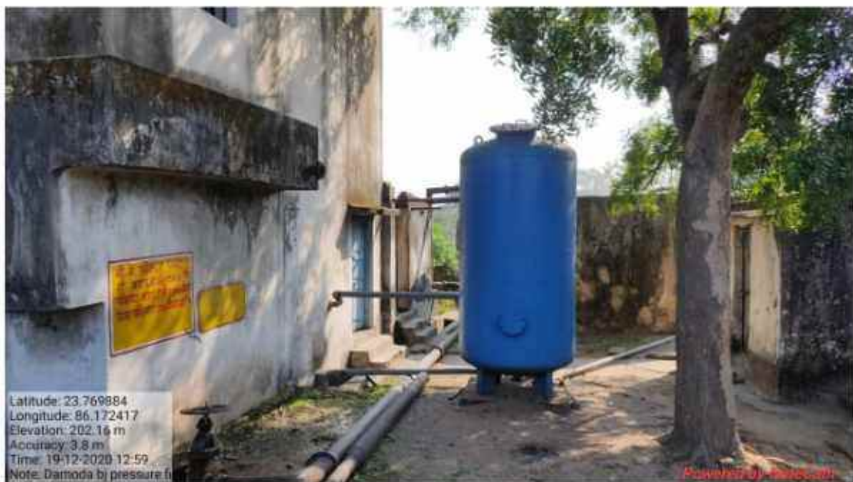
FILTER PLANT IN THE MINE AREA
