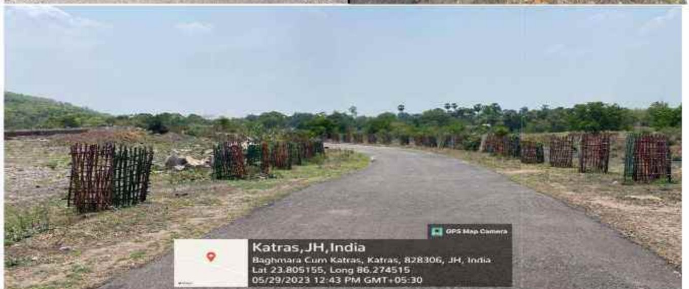
Bamboo gabion plantations along roads.
